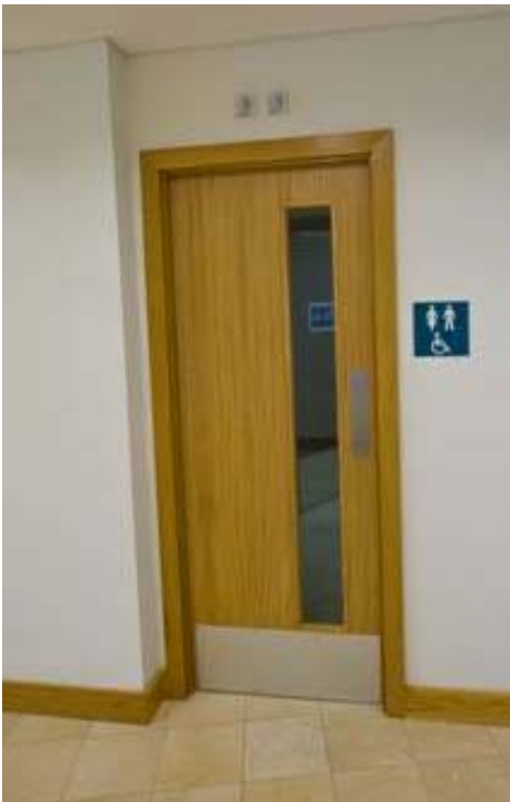
Figure 4 Internal Door and Sign
