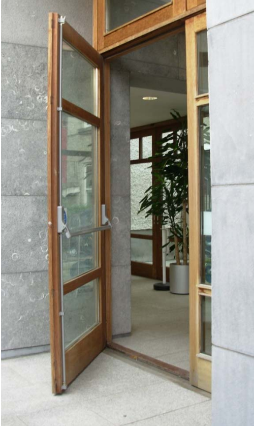
Figure 10 Emergency Escape Door
